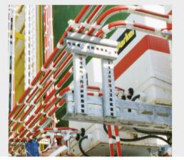
Heating of the impulse and sensing leads from the extraction point to the analyzing equipment
